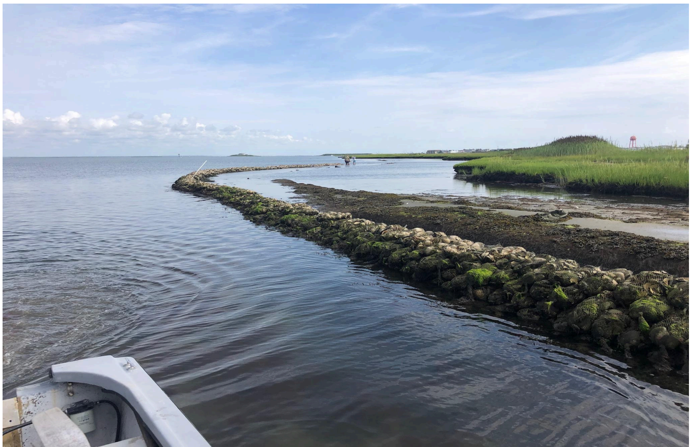
2024 view of western Mordecai Island showing oyster bags and backfill of sand and grasses.
