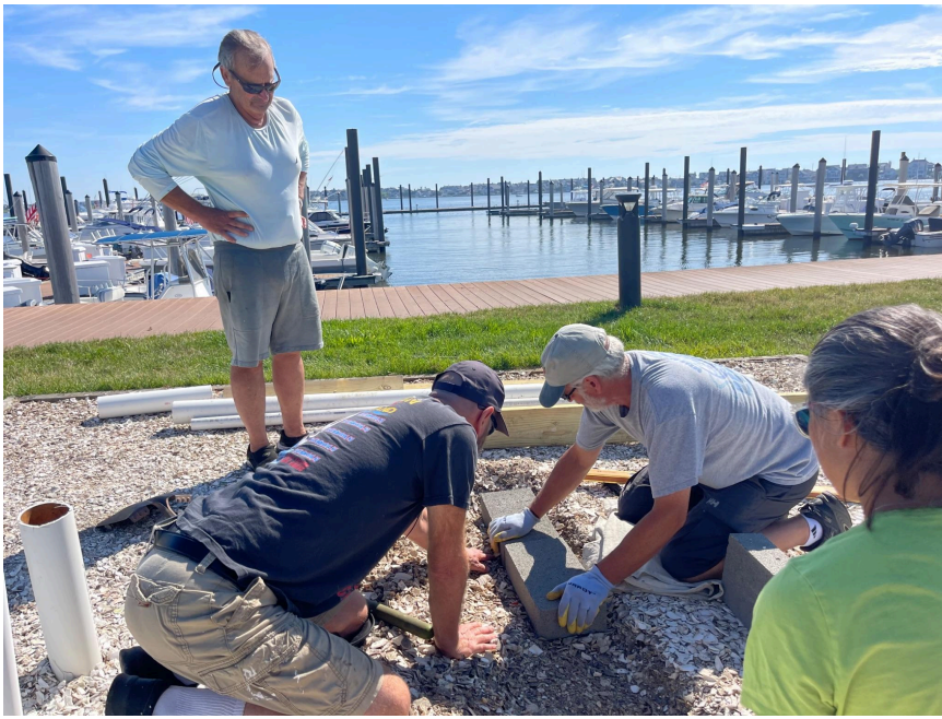
Laying the footings for the new Traders Cove upweller, 2024
