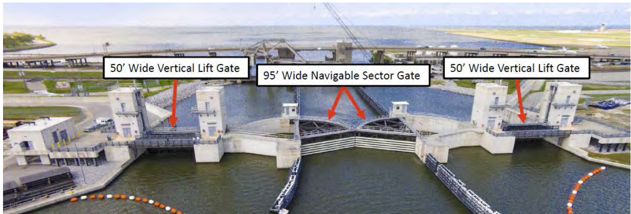
Figure 9-3: Seabrook Floodgate Complex
