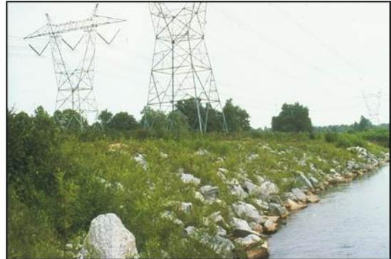
Figure 8: Typical Joint Planted Revetment
